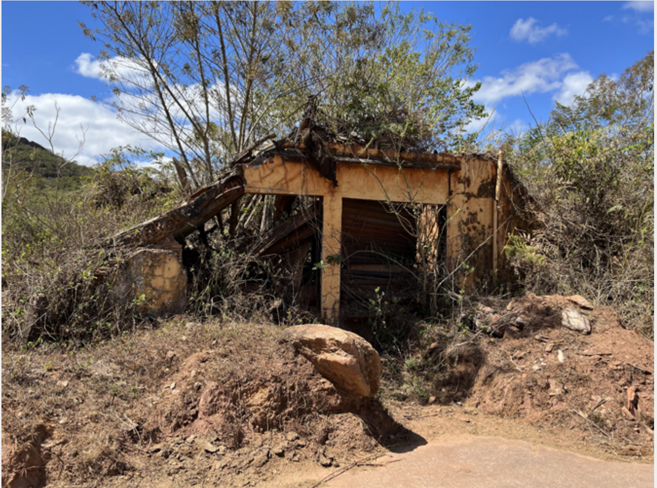
Structure destroyed by the Mariana tailings dam collapse, photo taken 27 August 2022
