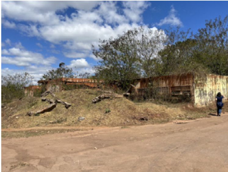
Mariana school covered in mud from the 2015 tailings dam collapse, photo taken 27 August 2022
